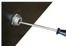
Once the temperature falls below approx. 75°C, the STL can be unlocked mechanically:
